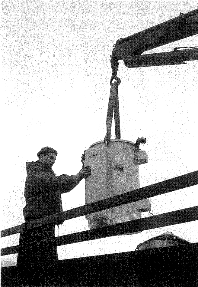
OP Recup 9 to 26 Jan 98 - Bdr Brain Brickell guiding a transformer in the back of an HLVW.
