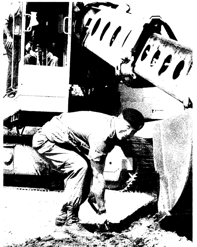
CO 1 RCHA, LCol Steve Gillies (with E Tool), and Base Comd CFB Shilo, Col Tim Guiler (with backhoe), break ground at the site of the new home for 1 RCHA - Aug 96.
