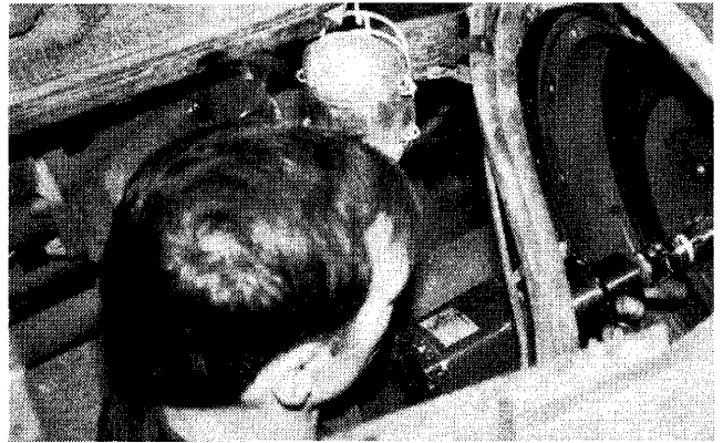
Second line repairs being carried out at 4 AD Workshop by MCpl Peloquin.
