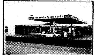
SERVICE STATIONS - Stations-service
