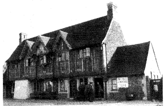
The Jolly Farmer, Runfold, near Farnham Surrey, Autumn 1940. Vestibule at left was built around one door to ensure effective blackout. Old inn sign preserved under glass at centre. Brick and stone work at ground floor is probably recent veneer over original half timber. Our party on right.
