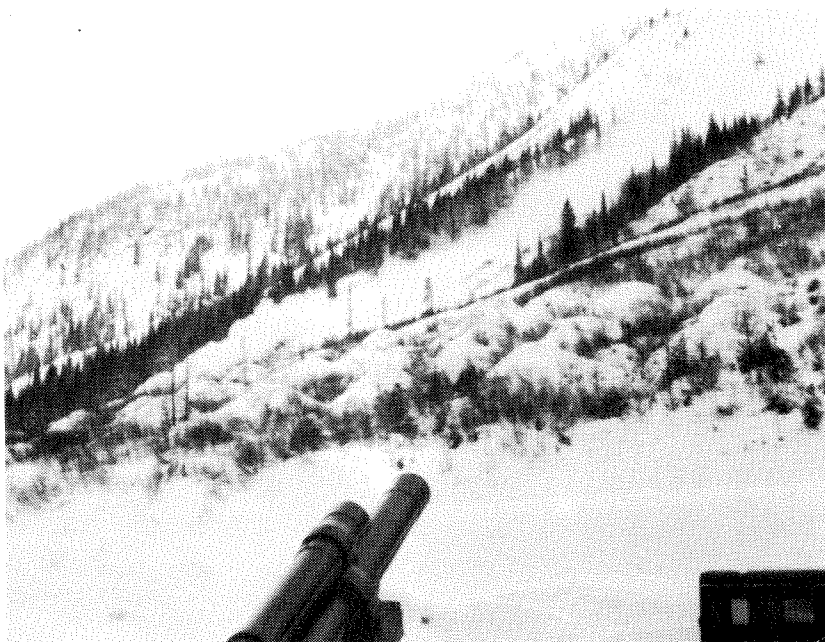
"The slides" momentum is broken up by the man-made earth mounds in the foreground.
