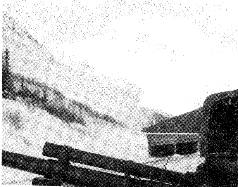
"Tupper Minor" Slide thunders over Lens Avalanche Shed on Trans Canada Highway.
