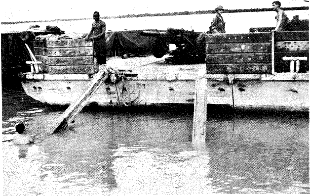
Bracing the barge with timbers for greater stability
