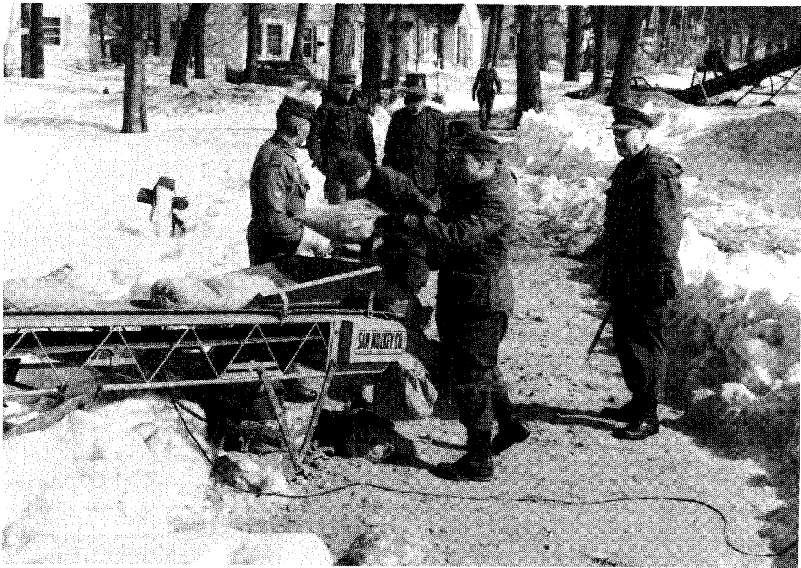
Mechanized sandbag operations at Elm Park dyke
