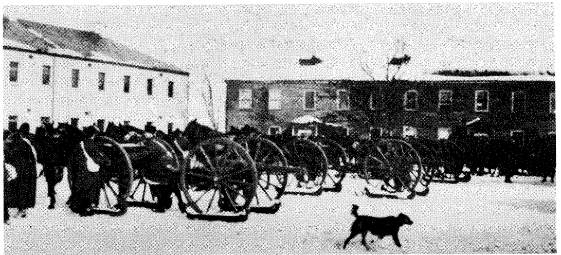
12 pr RBL guns on skids 1910 at Tete du Pont Barracks (now Fort Frontenac) Kingston, Ont. The wooden building in background has been replaced by a stone structure containing Staff College class-rooms.
